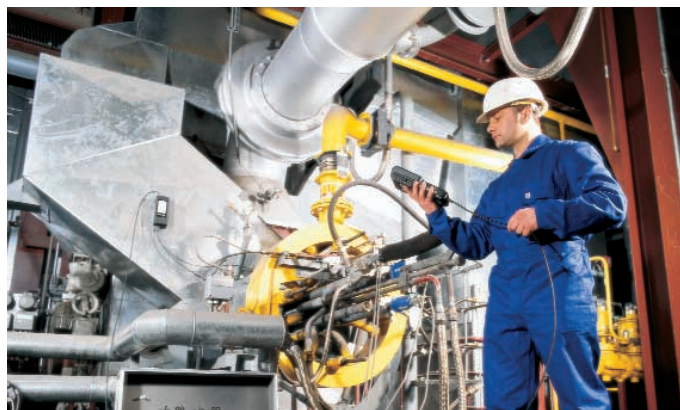
testo 350 XL: Standard set for measurements on process systems (O 2 , CO, NO, NO 2 )
